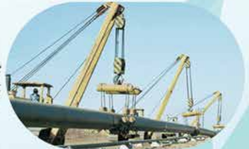
AME PIPELINE WORK PROJECTS
