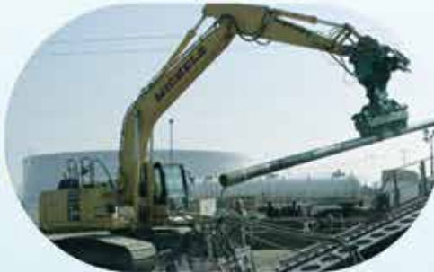
HORIZONTAL DIRECTIONAL DRILL
